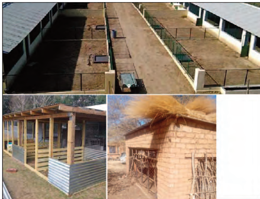
Figure 6.10 Walled and Roofed goat pens
