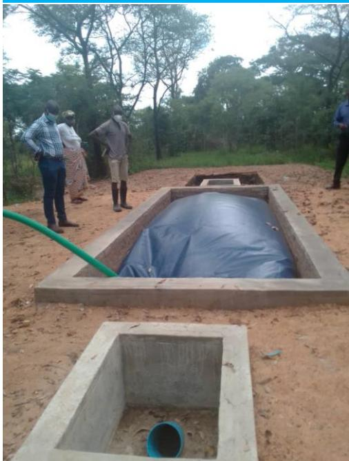
The biogas systems are to be fed with waste daily to avoid any glitches in functionality. Waste fed includes any bio-degradable waste around the household and other livestock waste including chicken waste. The biogas systems have a heating capacity for 5 000 chickens.
